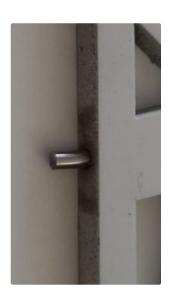
In the case of multi-part elements made of MDF and OAK PLYWOOD, Lamello connectors can be milled into the panel joints. A depth of 12 mm is required on each side for the milling. The pattern has sometimes to be adjusted slightly at these points.
